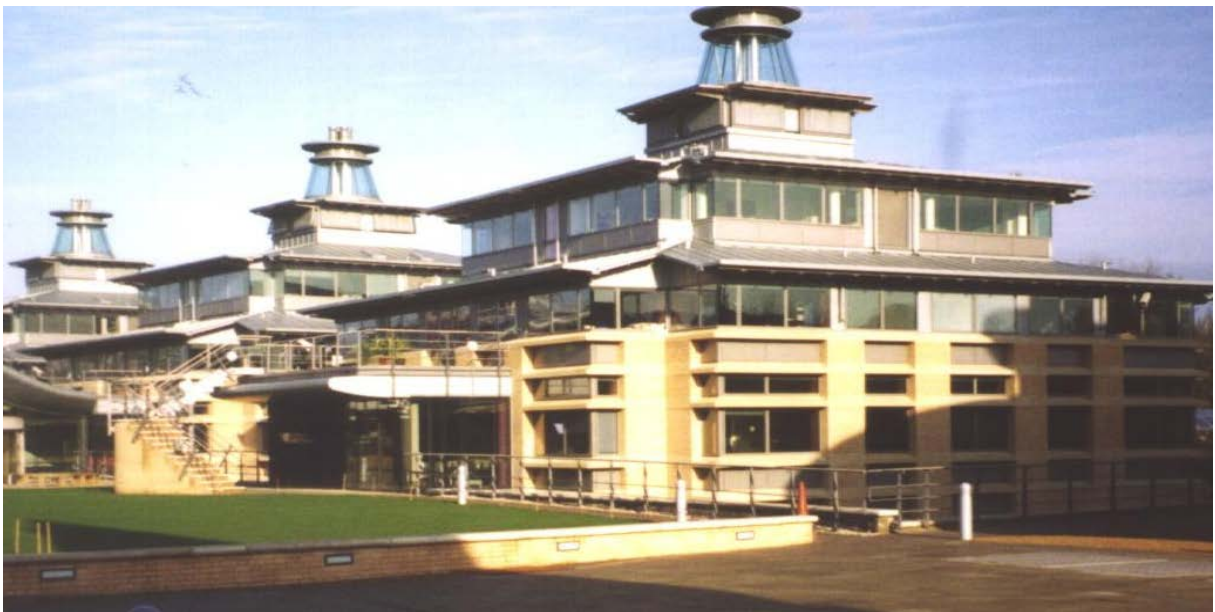
The Faulkes Institute of Geometry, completed in January 2002
