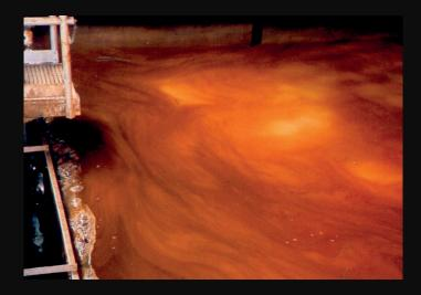
Dissolved air flotation tanks in one of Yorkshire Water's treatment works. The chocolate-like brown scum on the top is a foam comprised of the particles and the bubbles.
